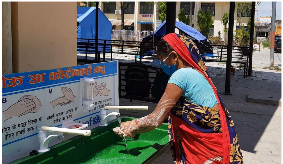
A service seeker at the Janakpur Provincial Hospital in Dhanusha District in Nepal's south washing her hands at the prefabricated handwashing station designed and installed by UNICEF. ©UNICEF Nepal/2020
